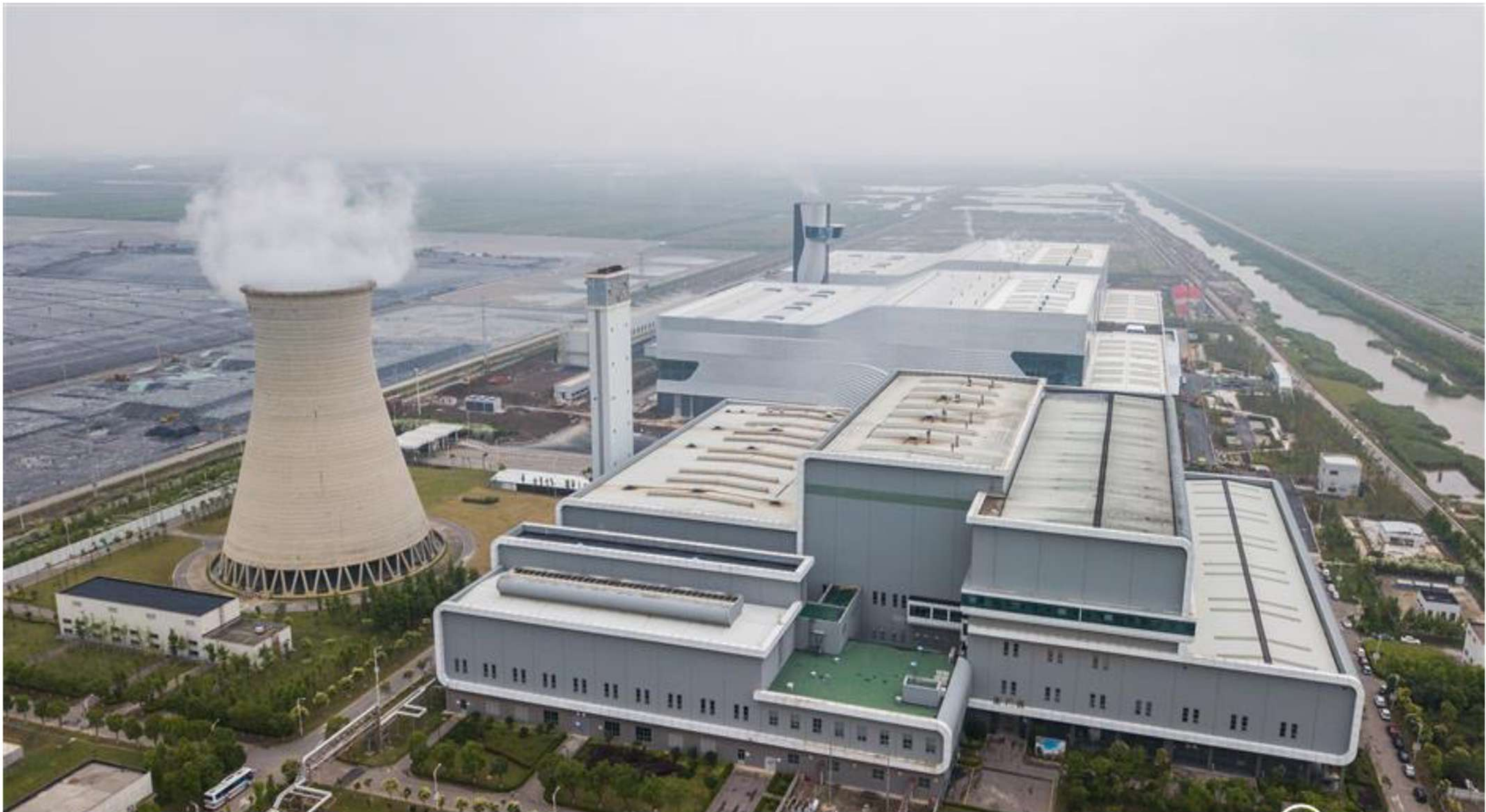
Shanghai Laogang Landfill Gas, China
