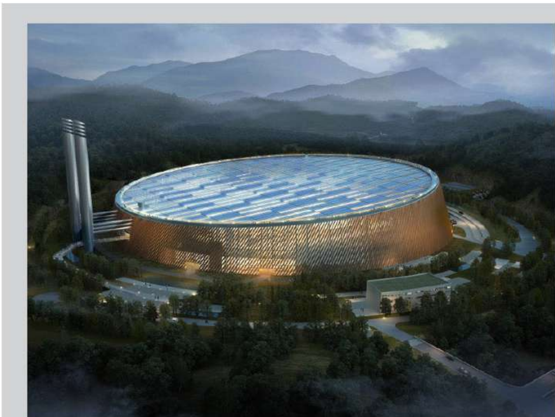
Sheznzhen WtE Plant
